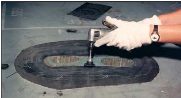
Figure 2 Manual removing of defected plies
