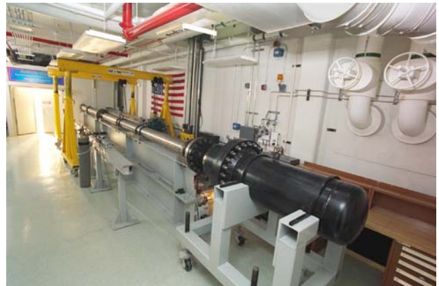
Fig. 9. GRC Ballistic Impact Facility.
