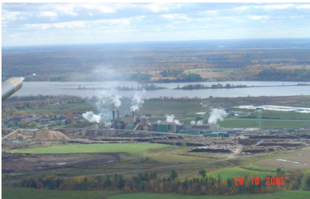
Fig. 9 Overflying the Thurso Paper Mill Smoke Stacks
