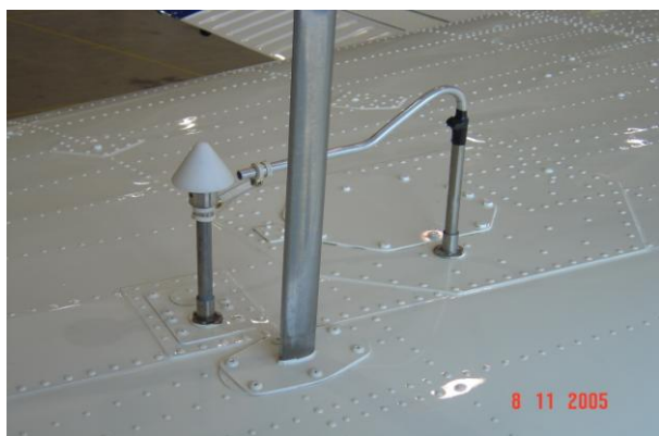
Fig. 12 Rooftop Gas Discharge-Inlet System
