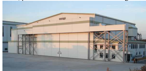
Fig. 2 External view of ETF showing main vehicle door in closed position
