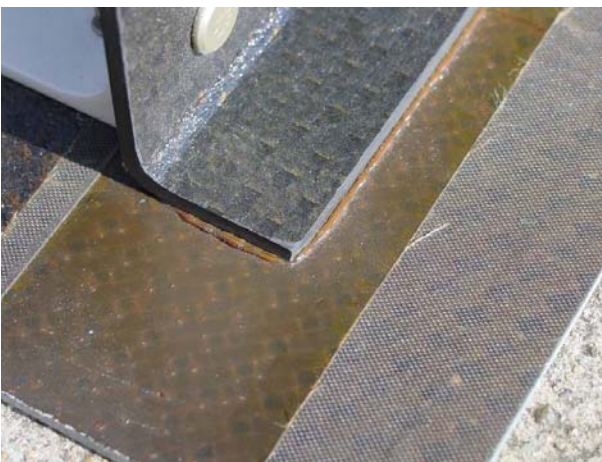
Fig. 10. Close-up of Welded Joint
