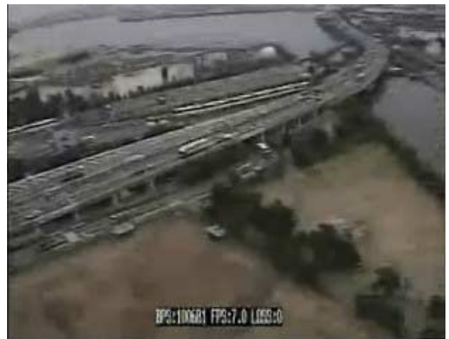
Fig. 10 Video Image Transmitted Using Cellular Phone Data Link System
