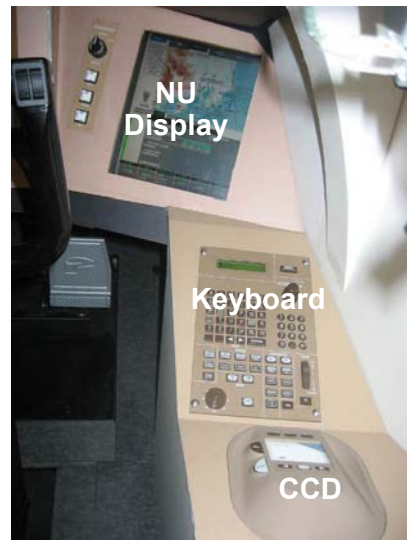
Figure 14. Navigation Unit System Installation
