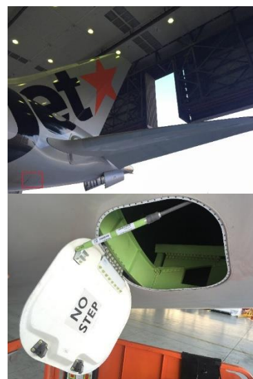
Fig 3: Location of access hatch on 787-8 aft of the rear pressure bulkhead
