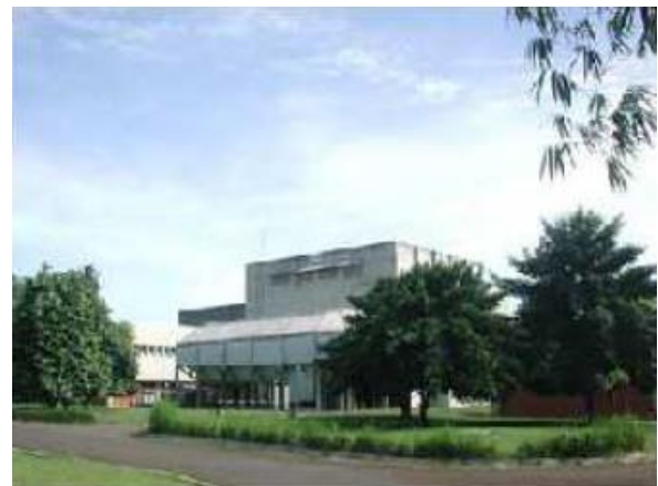
Fig. 1. Indonesia Low Speed Tunnel.
