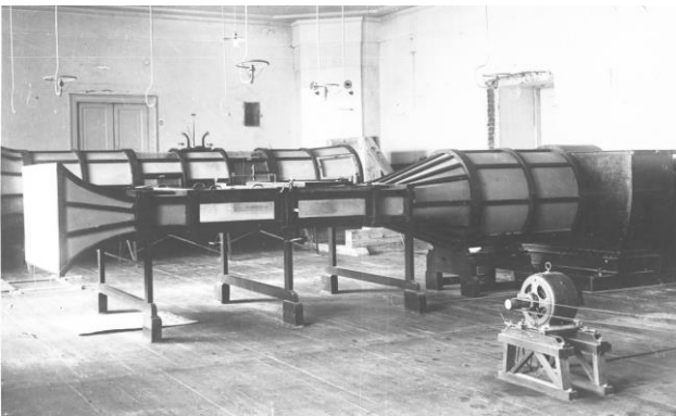
Fig.10. Photograph of two wind tunnels of the Imperial Technical School
